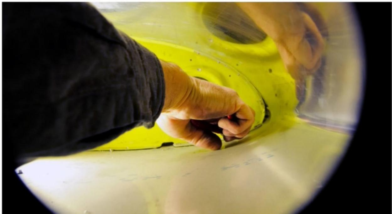
This entailed more than just drilling out hundreds of rivets, however—throughout the process, he was looking for clues as to how the wing originally was put together, to guide him in the eventual reassembly. The service manual doesn't provide step-by-step instructions for a project like this; Young and his co-workers were on their own.
